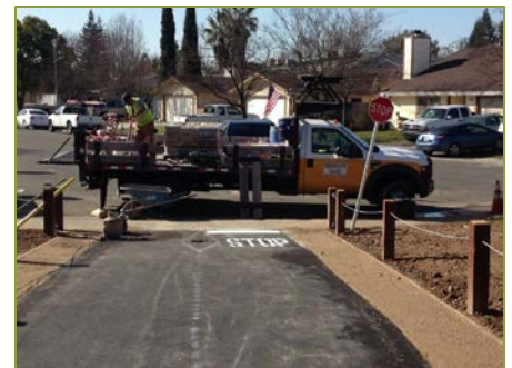
Image of trail construction in Elk Grove.
