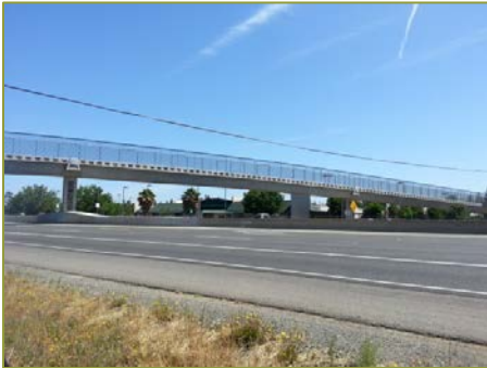
Image of the newly constructed pedestrian bridge over Highway 99
