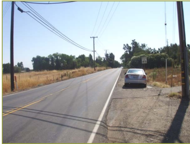
Constructing bikeways and trails in correspondence with road construction projects.
