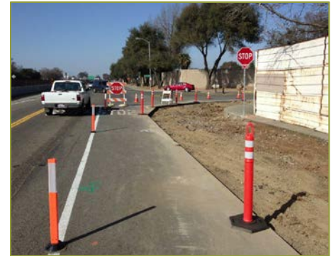
Sidewalk infill construction in Elk Grove
